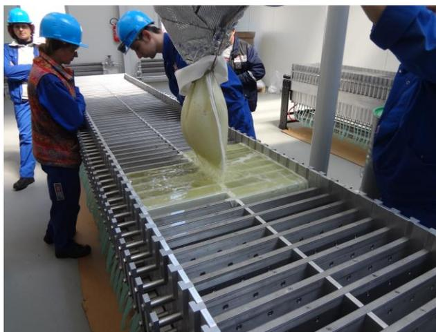
7. If using the same filter bag, for multiple pouring's of wax, verify that the bag is not solid with wax.
